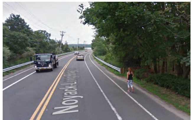
Noyac Road in Southampton has bike lanes and a narrow paved area for pedestrians with pinch points at bridges, but lacks sidewalks
