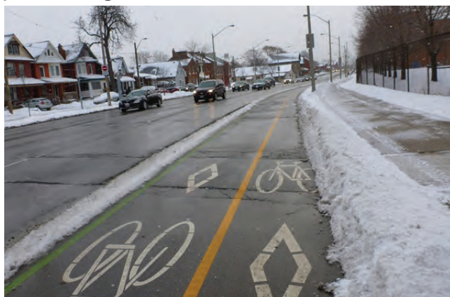
Figure 65: Hamilton, ON – Two-way cycle tracks in Hamilton are routinely cleared of snow using plows (Image: Norma Moore)
