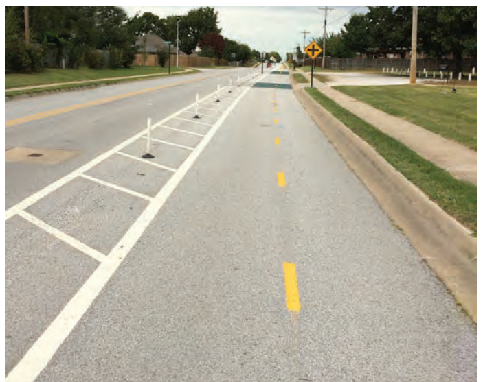
A two-way, separated bicycle facility in Arkansas (Image: EST Design Guide)
