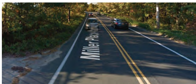
Figure 29: Insufficient Width for Shoulders and Bike Lanes
