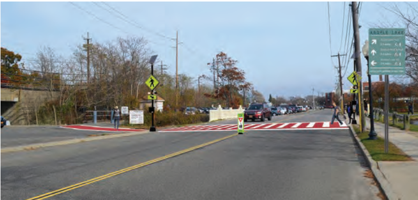
Figure 7: Photo simulation illustrating a mid-block crossing with Rectangular Rapid Flashing Beacons and a crosswalk extension to a pedestrian underpass beneath the rail tracks on Trolley Line Road in Babylon
