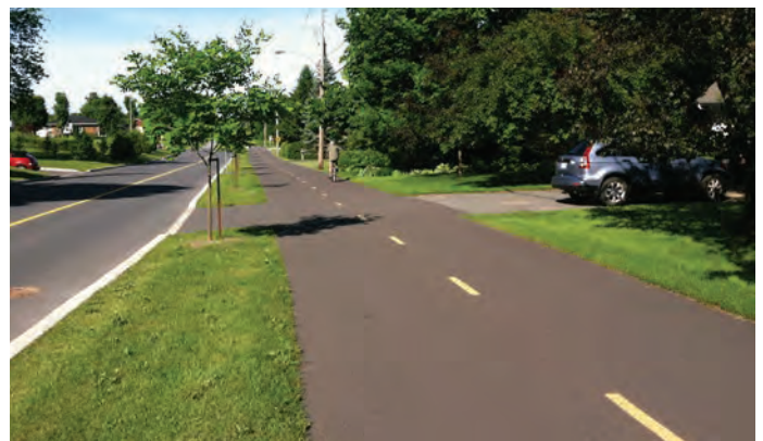
Rue Drumond in Granby, Quebec features a typical sidepath, separated by a landscaped area. The sidepath has priority over driveways and minor intersections. Motorists must yield to pedestrians and bicyclists on the facility.
