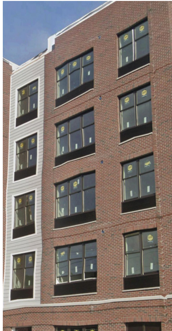
Through wall units integrated into window composition
